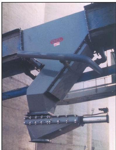
Aerated lump trap with slide gate valve.
