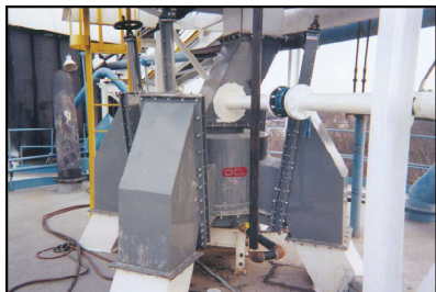
Aerated distribution box with four discharges.
